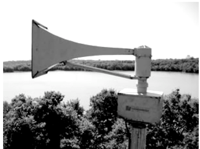
Figure 2. A siren as an outdoor warning noise-maker.
